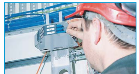
A WH Electrical technician terminating fibre optic cables.
