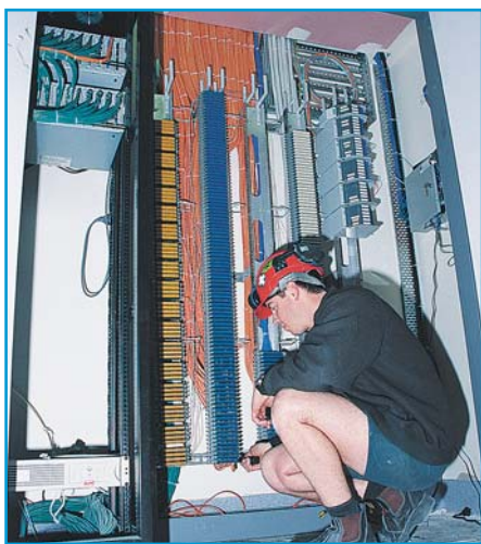
Terminating Clipsal 3100 Modules using Clipsal IDC Termination Tool designed to provide reliable connections.
